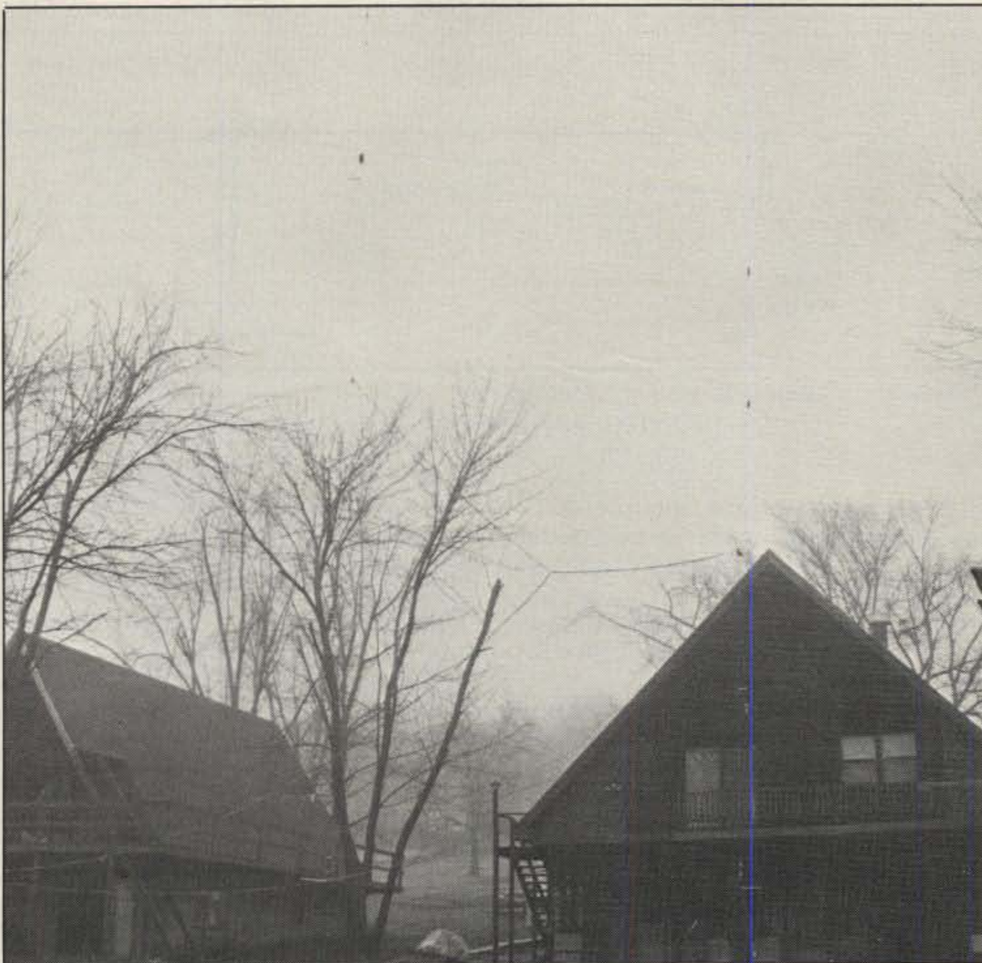
The all-band phased array installation at KAØRUM. The top support is nylon rope stretched between the tops of two high trees. The bottoms of the dipoles are weighted by concrete blocks with screen-door springs to relieve wind stress. Feedpoints are held apart by additional nylon cords pulling away from the center of the array.
